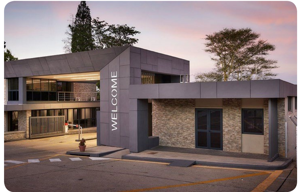
* Main entrance to Mintek in Randburg, South Africa.
